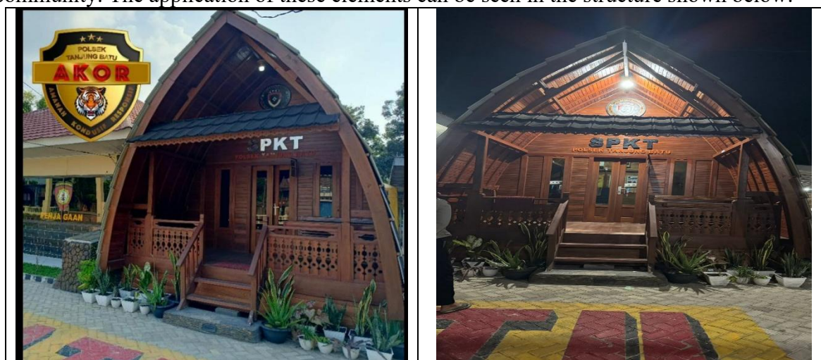
Figure 1. SPKT Building of TJ Batu Police Station
